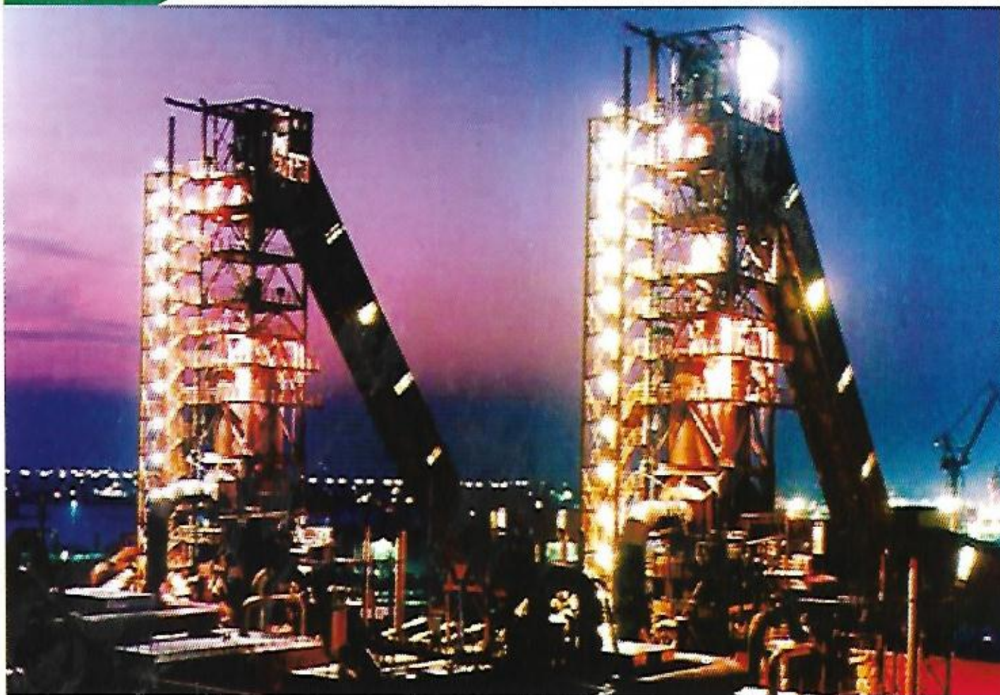
Fig. 3: Direct Reduction Modules after commissioning
