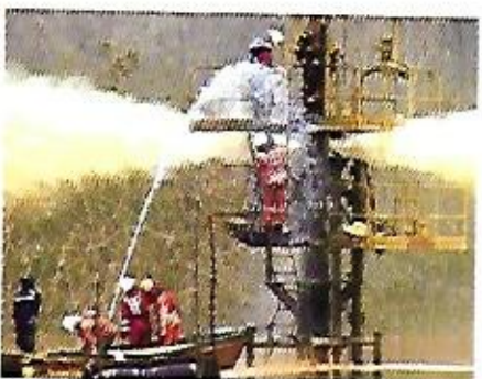
Fig. 12: Nembe oil spill contingency team working to repair the damaged wellhead
