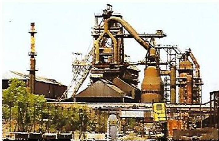
Fig. 4: Ajaokuta Steel Plant
