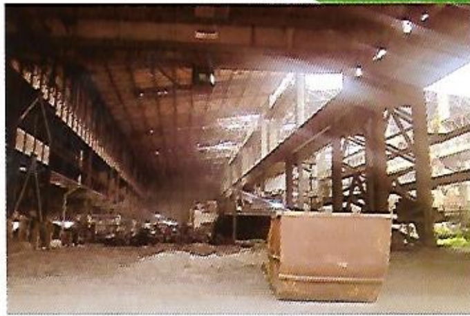
Fig. 5: Steel Melting Shop at Delta Steel Company
