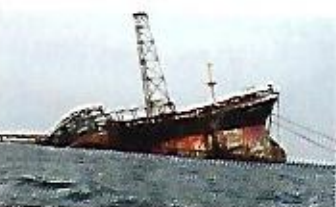
Fig. 15: SEPCO FPSO Accident; off the coast of the Niger Delta; during which reports say that oil spill was generated / discharged
